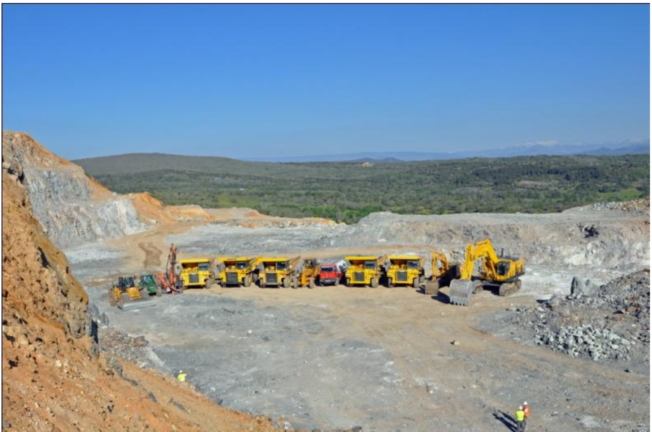
Figure 2: SyL's new mining fleet assembled in Los Santos South pit
