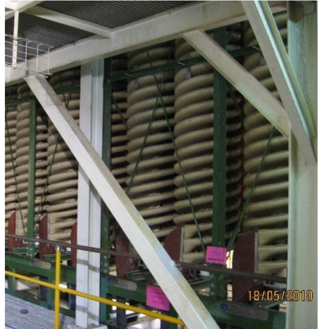
Figure 1: Newly installed spirals prior to commissioning
