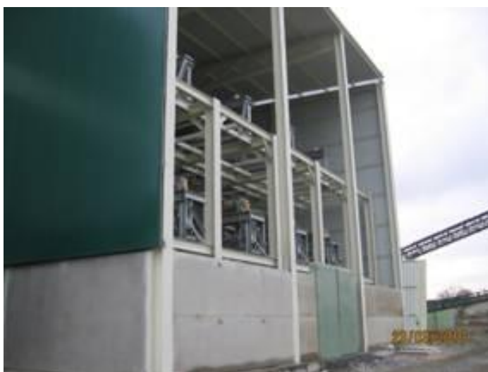
New Building Structure
