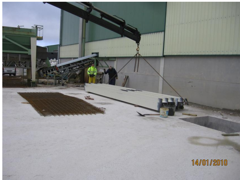
Figure 2: - Concrete base for additional Mill modifications completed.
