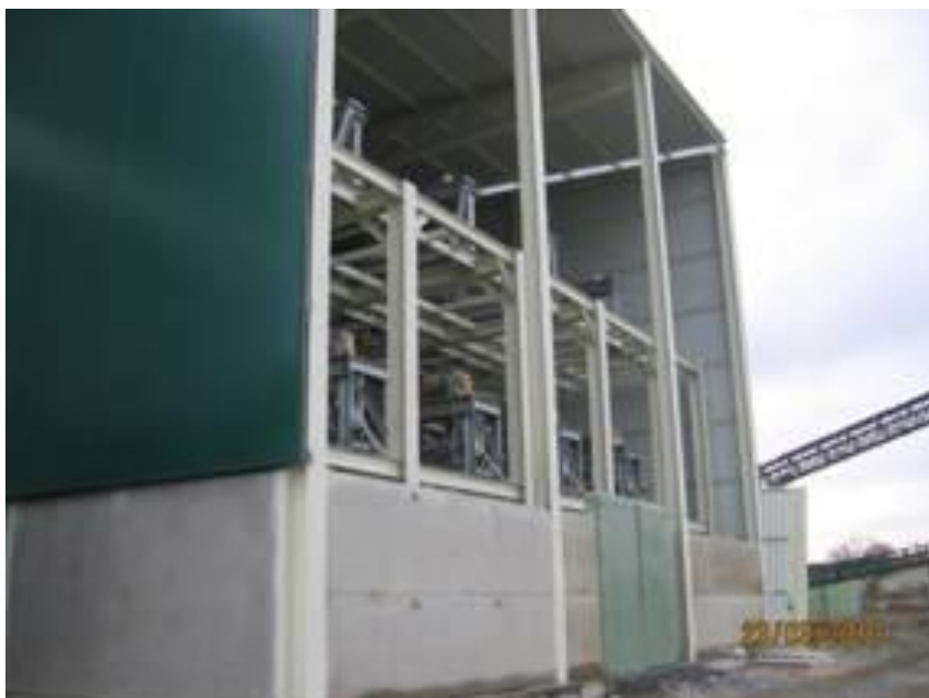
Figure 2: - New Building Structure at Los Santos housing additional tables
